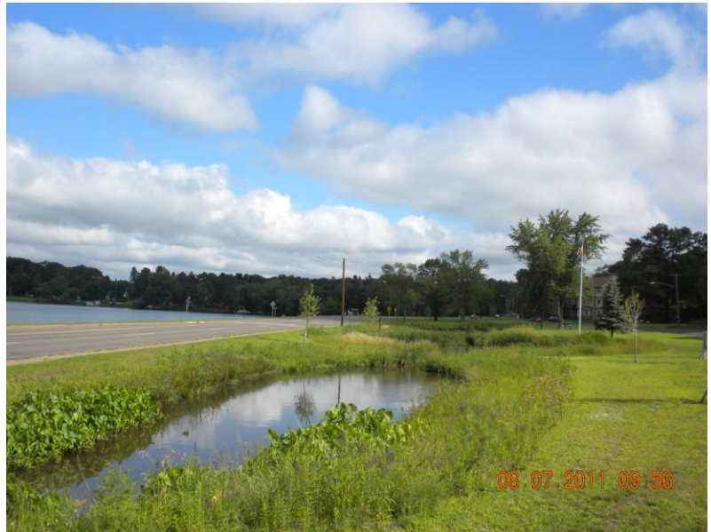
Figure 7. Flagpole Park Stormwater Wetland
