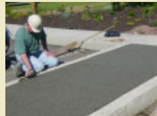
5. (above) Work edges and surface to a clean finish.
