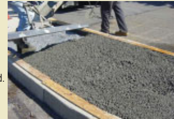
4. (above) Concrete is leveled with a screed.
