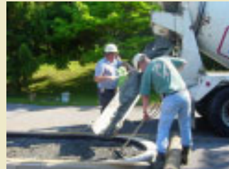
3. (above) Concrete is poured and spread.
